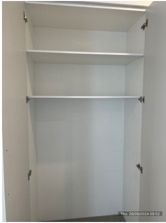
Landing: Built in cupboard (photo 2 of 2)
