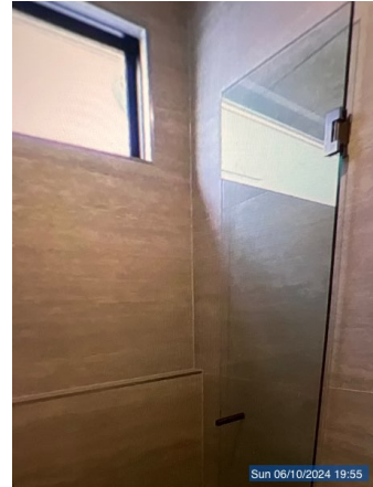
Ensuite: Shower/screen/taps (photo 1 of 1)
