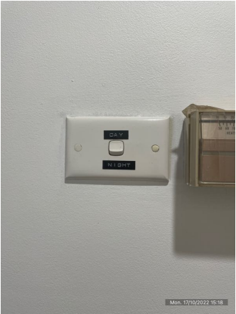
Entrance Hall: Old heater switches (photo 3 of 3)
